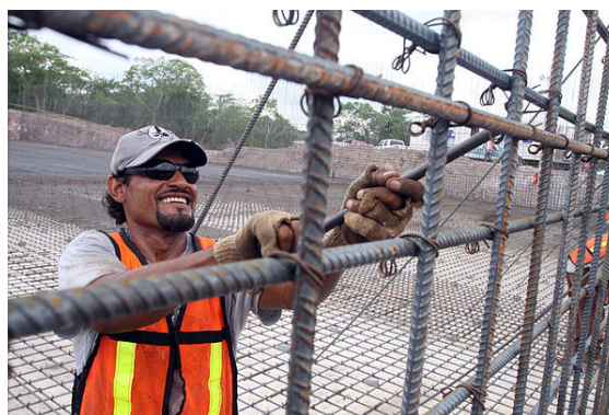
Worker assembling rebar for a water treatment plant in Mazatlan, Sinaloa, Mexico.
